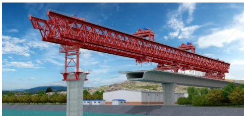
Gambar 2. 2 Erection Box Girder
